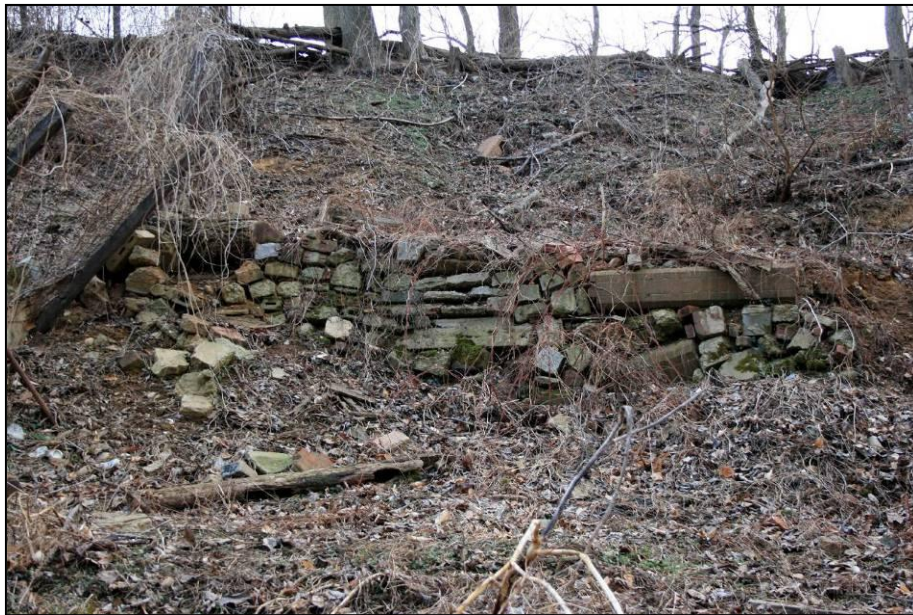
Figs. 149, 150: The stone wall on the West Slope.
