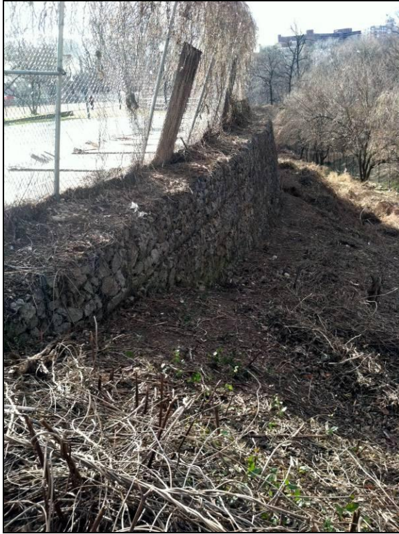
Figs. 40, 41: Two views of the gabion wall that separates the Upper Plateau of Walter Pierce Park from the North Slope. The construction of the wall in 1982 required deep footings, causing major disruption of the land on the North Slope. Water that seeps through the gabion wall from the Upper Plateau has contributed to erosion on the North Slope.
